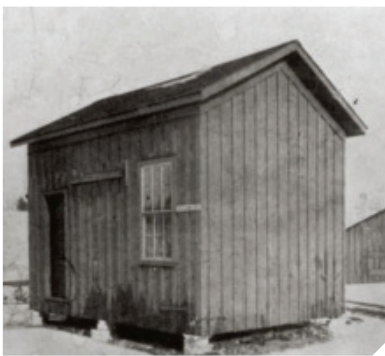
The original Vulcan Street Plant burned down. A replica was built in its place
