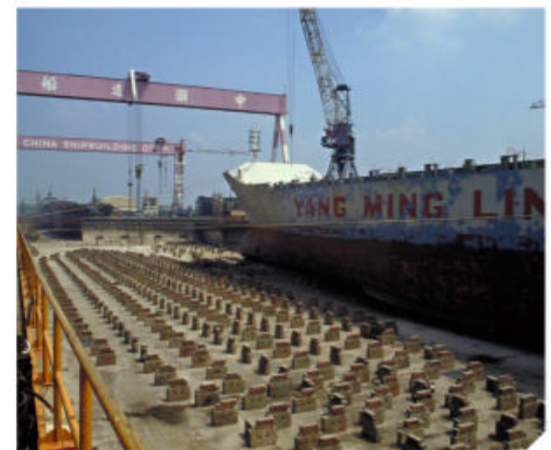
Kaohsiung dry dock is located in Taiwan's largest port
