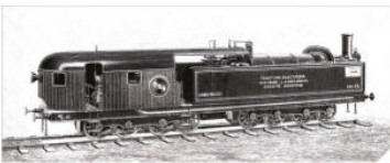
An illustration of one of Heilmann's experimental steam-electric locomotives
