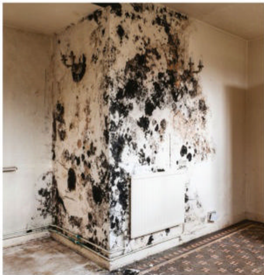
It can take less than a day for black mould to appear on damp walls
