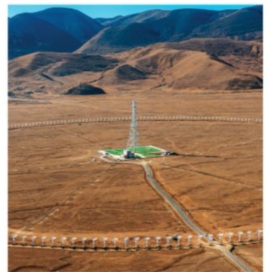
An aerial view of the construction site of the Solar Radio Telescope in Daocheng County, Sichuan Province, China
