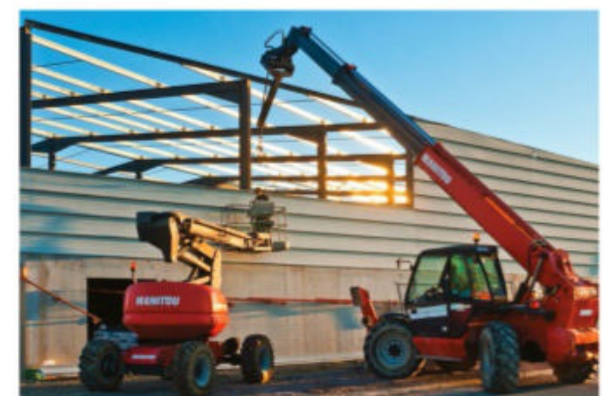
Mobile cranes are usually used to erect steel structures and unload ships.
