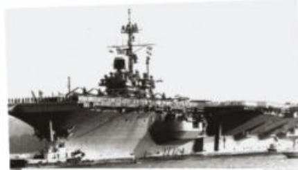
The USS Ranger was the only carrier in its class and was the first to be built from the keel – the ship's structural beam – up.
