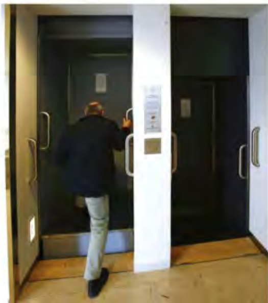
A man steps onto a moving paternoster as it travels upwards. The right side is moving downwards
