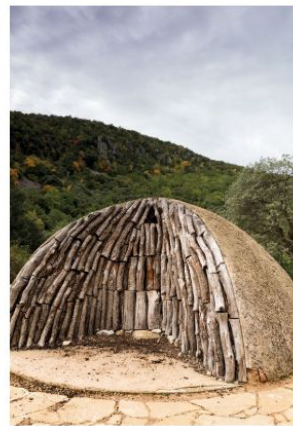
Ancient charcoal ovens burned wood under clay to keep air out
