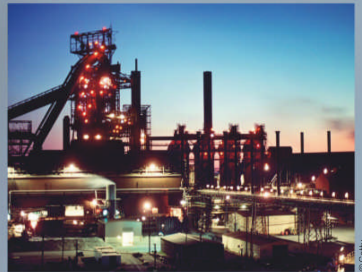
Pipes circulate gas around blast furnaces to help produce molten iron
