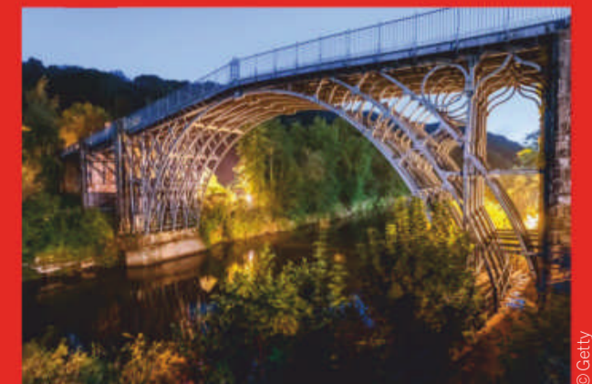
Ironbridge in Shropshire, England, was made possible by using coke in blast furnaces
