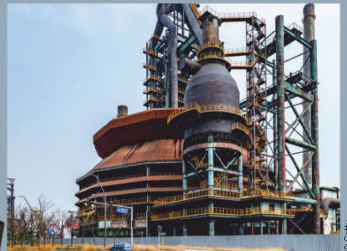
As rocky pellets fall into a blast furnace, hot air from below sets them alight
