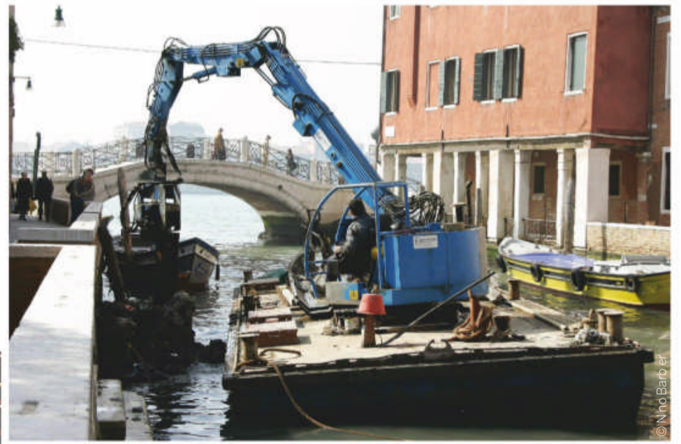
A floating excavator dredges debris from one of Venice's canals
