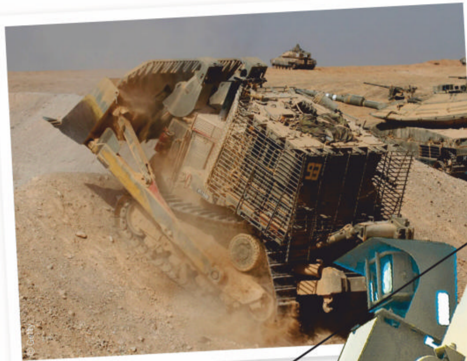
The IDF Caterpillar D9 is clearing the path for battle tanks by moving the earth
