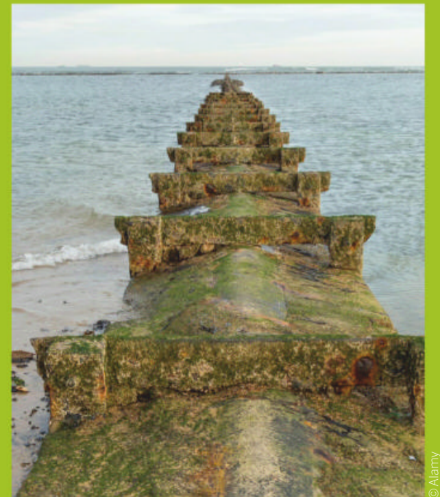
Some wastewater systems can't handle the large volumes of storm sewage, so this water often bypasses in large pipes
