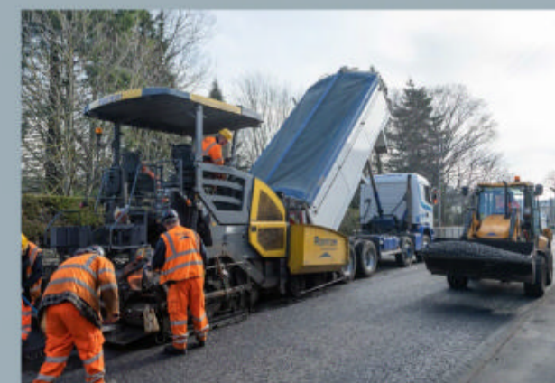
Road layering taking place with a recycled plastic and asphalt mix
