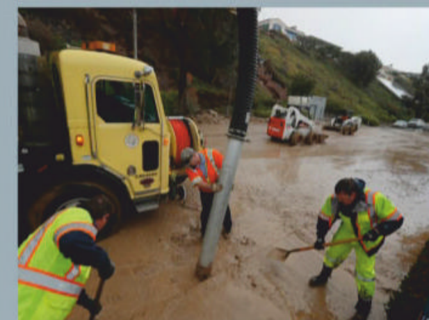
Hydrovacs helped clean up the debris from a landslide in California in 2018
