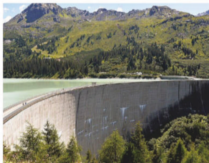
Before building a dam, the river has to be diverted to keep the construction site dry
