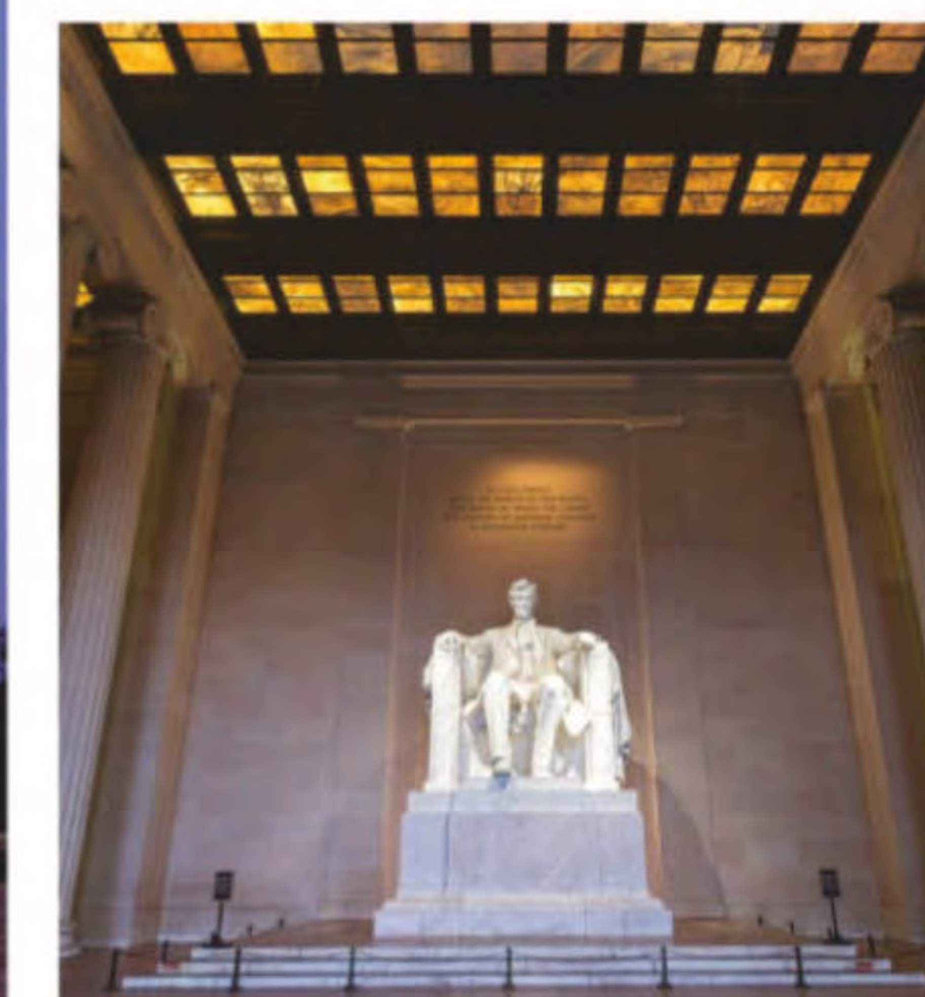
The ceiling tiles were made from Alabama marble and soaked in paraffin to turn them almost translucent
