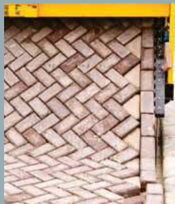
Road printers are the fastest and most reliable way to build a brick road
