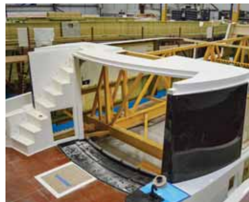
Above: While the hull is being finished the upper decks are being built almost simultaneously
