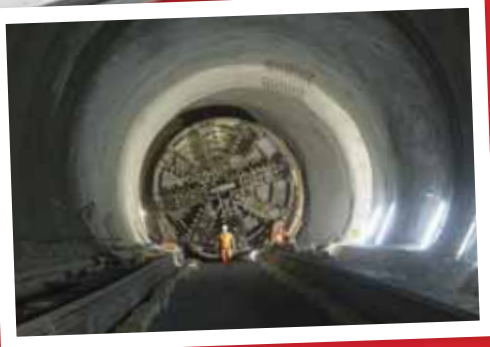
Crossrail's TBMs carved out approximately 3.4 million tons of earth over three years
