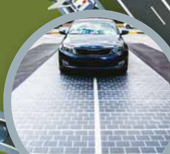
The Wattway was installed at the West Point Visitor Information Center in 2016
