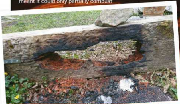
The fire burnt slowly for several days because a lack of oxygen deep in the wood meant it could only partially combust
