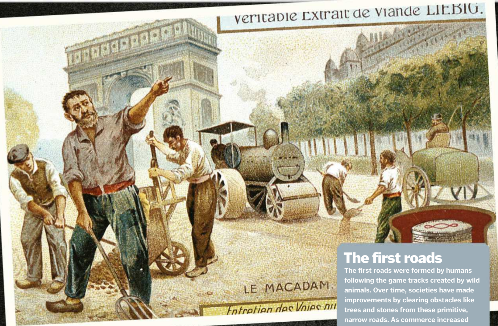
Laying a macadam road surface involved compacting the road covering with a steam road roller
