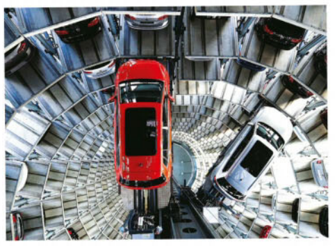
The Car Towers are recognised as the "fastest automatic parking system in the world", moving vehicles at speeds of 2m/s
