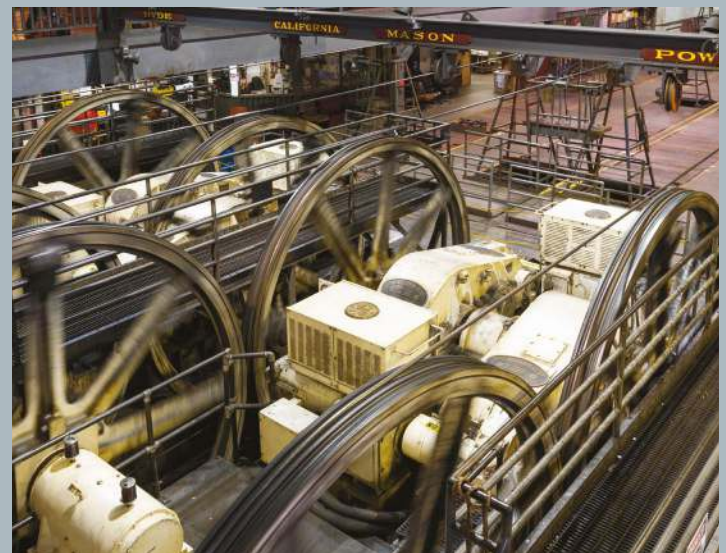
Large wheels drive the cables from inside the powerhouse
