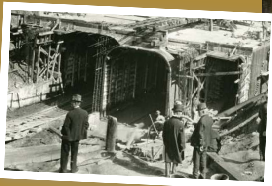
The twin tunnels of the Cincinnati subway, under construction in the 1920s
