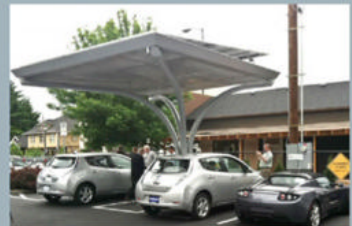
This solar panel parking unit was installed at a parking lot in Portland, USA, in 2011 for electric cars to use
