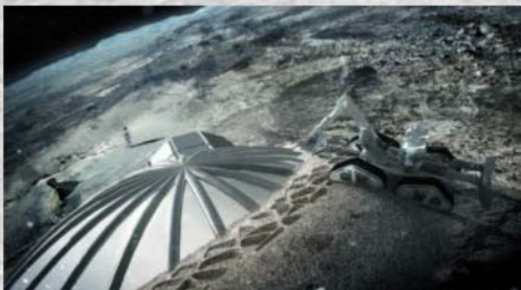
The 3D-printed shell is made up of a hollow closed-cell structure - reminiscent of bird bones
